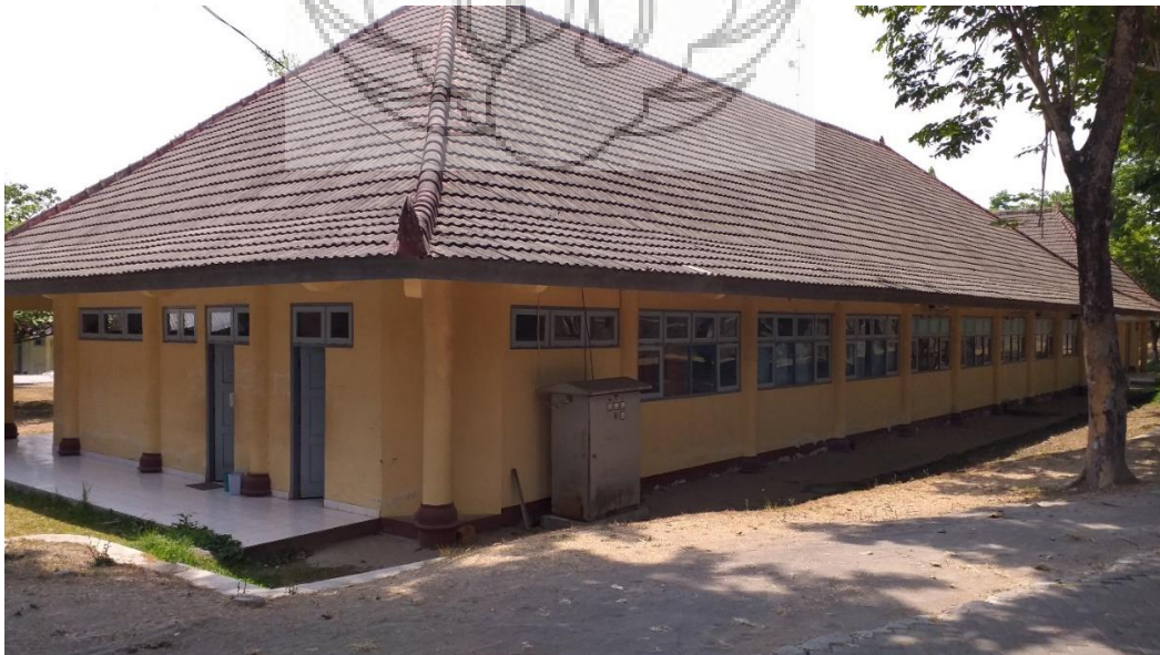
Gambar 2.28 Existing Tampak Samping Gedung 5
