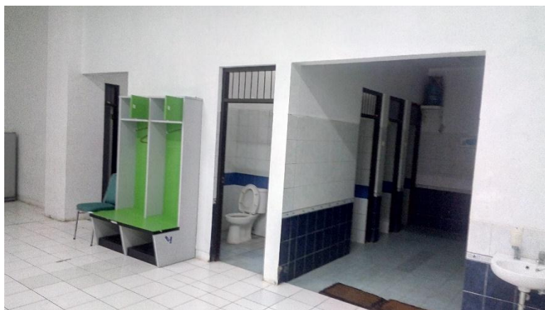
Gambar 1.5 Shower Ruang Ganti
