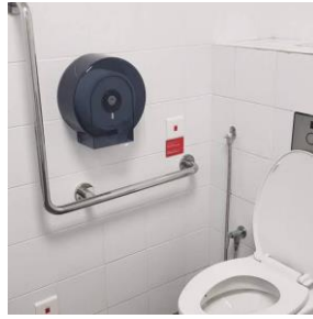
Gambar 5.8 Tombol Emergency (Sumber: https://www.ipsec.com.my/products/building , 2023)
