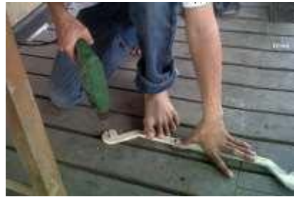
Picture. 38 process of installing the Kesok-kesok friction rope
