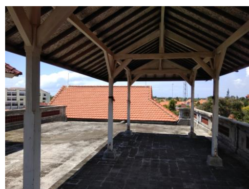
Gambar 7. Rooftop (Sumber: Marina Armedia, 2017)
