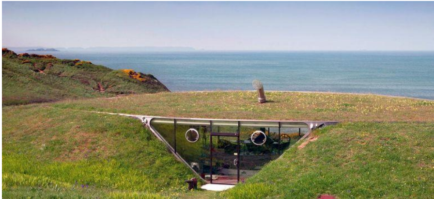
Malator house(Architecture UK/Alamy)
